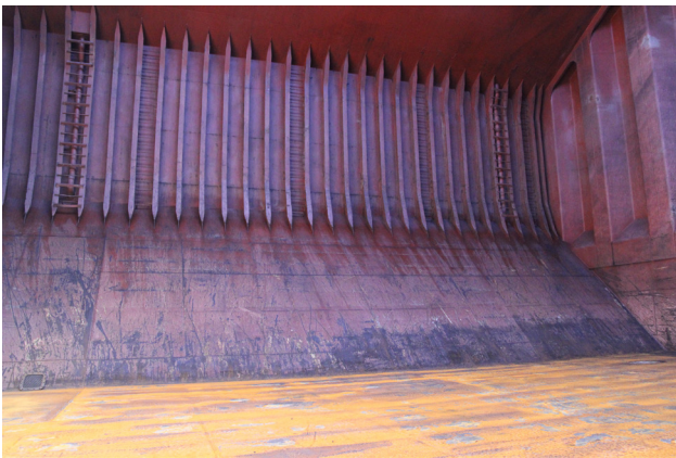
Figure 2. Deteriorated paint coatings provide cargo stains good adhesion to the surface into the pores. It gets progressively more difficult to clean off too.
